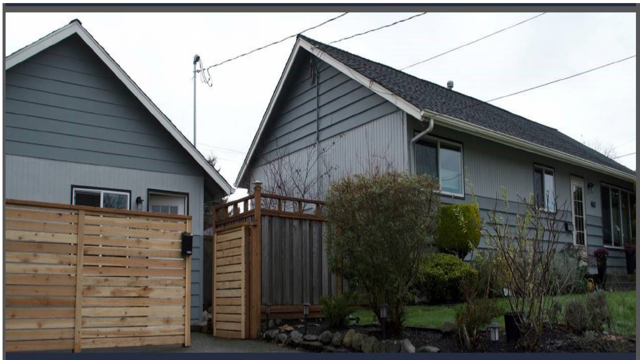
Converted garage Detached ADU - 2019
